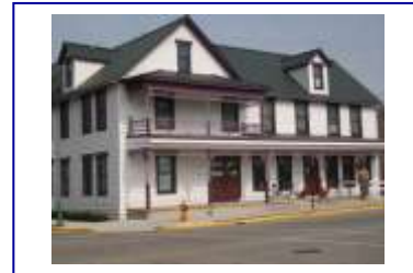
← Whitewater Hotel Restoration
