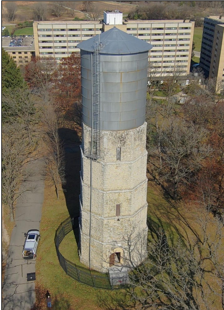
Photo 1: Starin Park Water Tower
