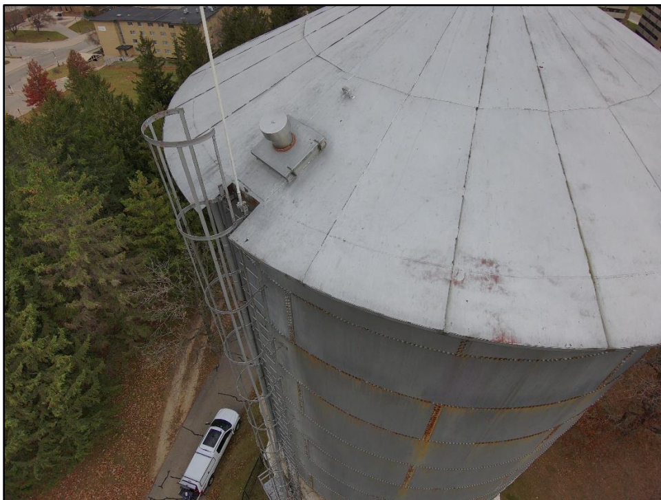
Photo 9: Exterior ladder to tank
